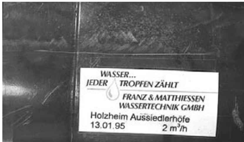
Picture 4: longitudinal tear in PVC-pipe
